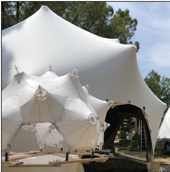
Figure 24: Left (Top): Placing Membrane; Left (Bottom): Original design in 1:6 mockup with the final build 1:1 dome; Right: Fully stretched membrane. (photos by: Uri Lewis)
