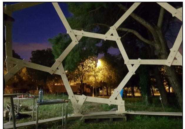
Figure 21: Assembling 3 rd row structure planks.
