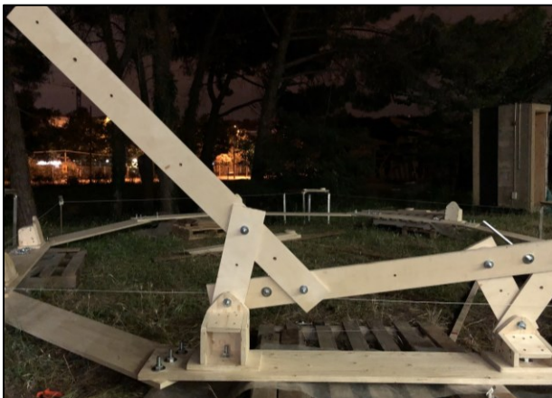
Figure 20: Assembling supports and 1 st row planks.
