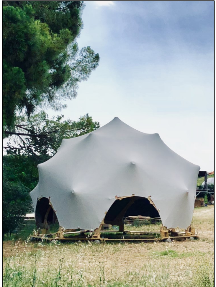
Figure 24: Left (Top): Placing Membrane; Left (Bottom): Original design in 1:6 mockup with the final build 1:1 dome; Right: Fully stretched membrane. (photos by: Uri Lewis)
